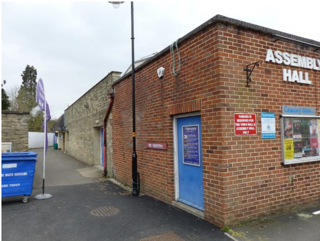
Photograph 3: Left hand elevation.
