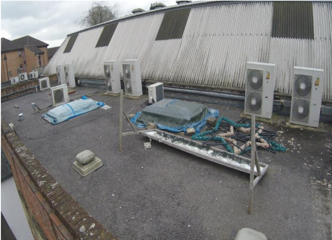
Photograph 19: Front centre flat roof.
