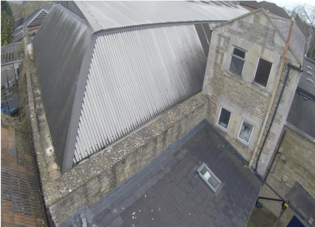
Photograph 7: Right hand elevation of the three storey section.
