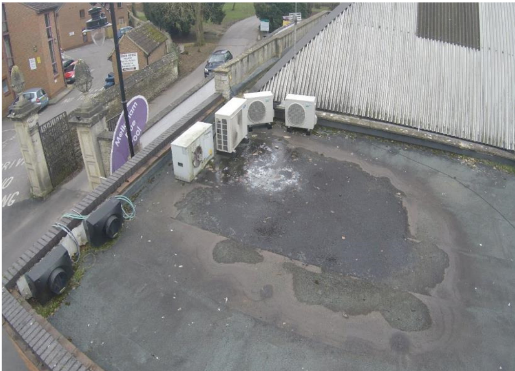
Photograph 16: Front left hand flat roof.
