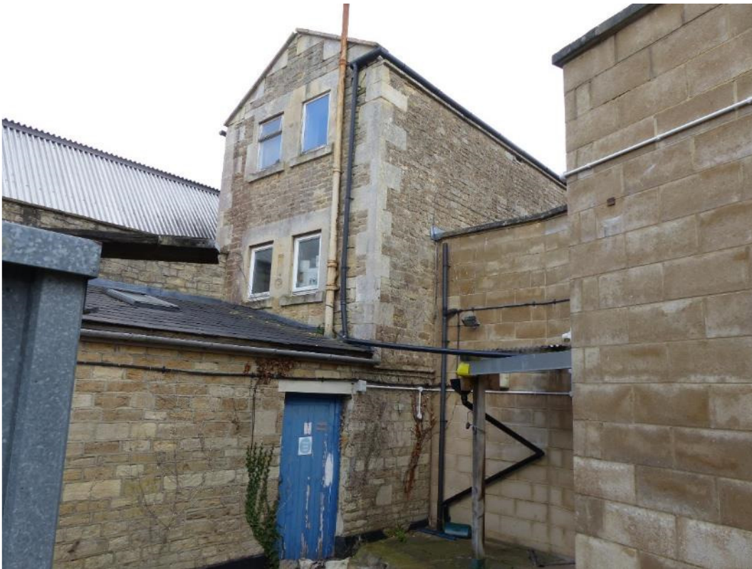
Photograph 29: Rear right hand fire escape. Note downpipe from three storey section.
