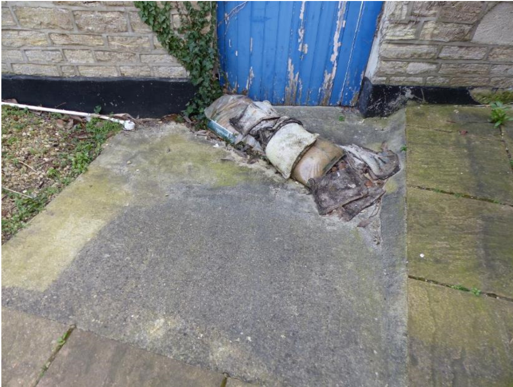
Photograph 35: Well area and sand bag outside the rear right hand fire exit door.
