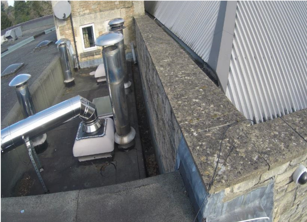
Photograph 23: Roof over the boiler room.
