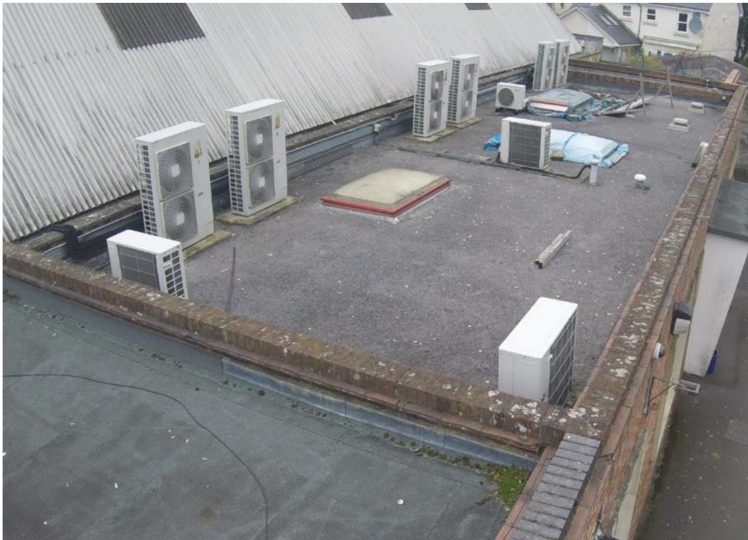
Photograph 18: Front centre flat roof.
