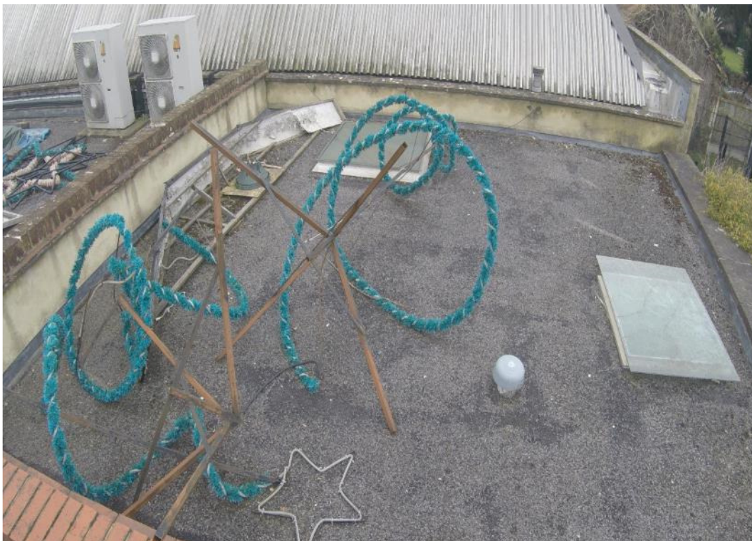
Photograph 20: Front right hand flat roof.
