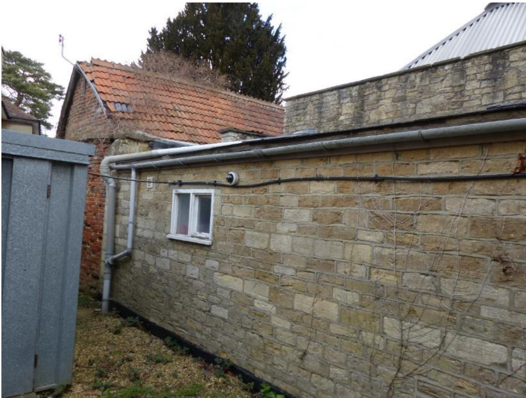
Photograph 9: Rear elevation of the right hand side.
