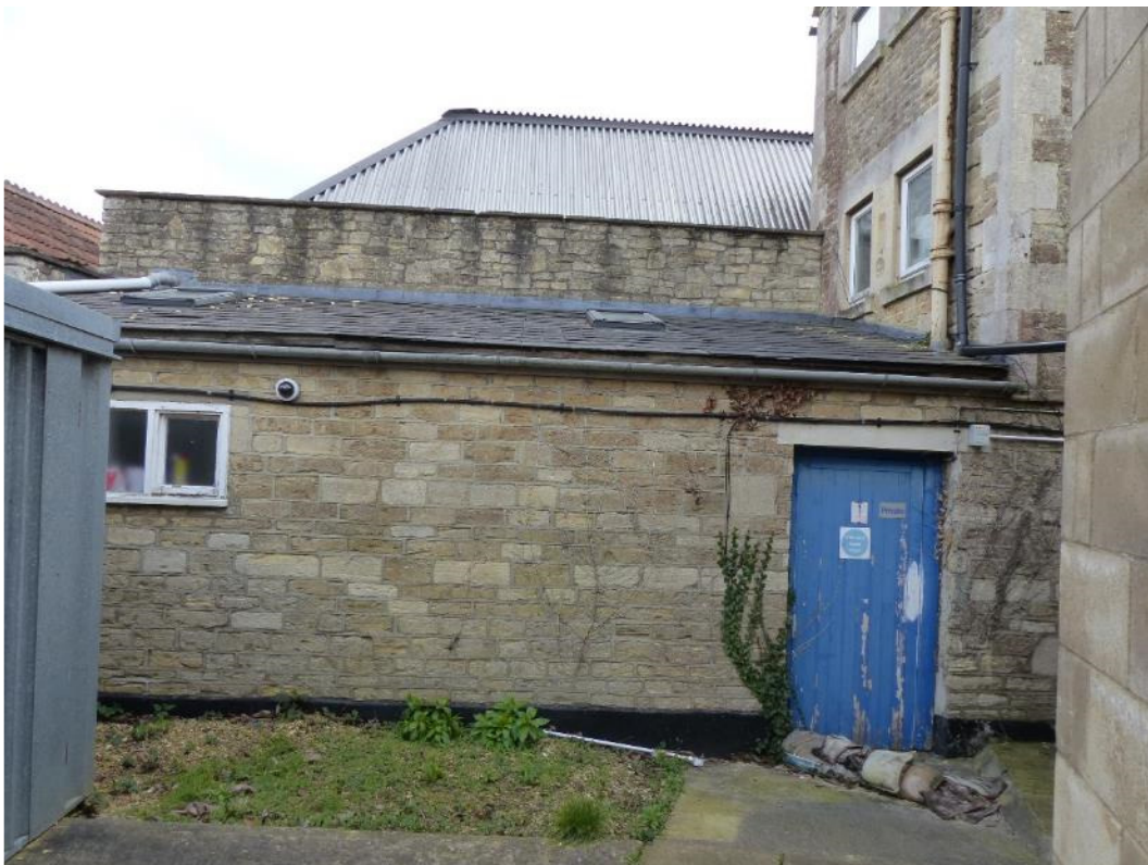
Photograph 8: Rear elevation of the right hand side.
