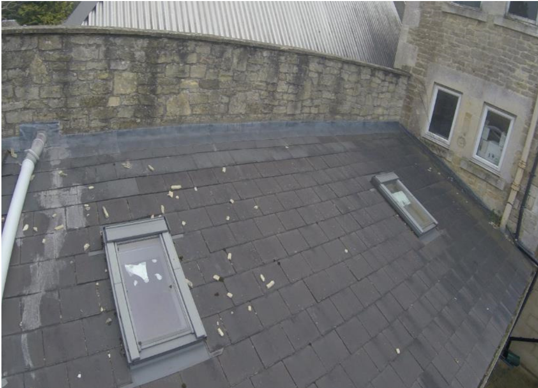
Photograph 25: Roof over the rear right hand office and laundry area.
