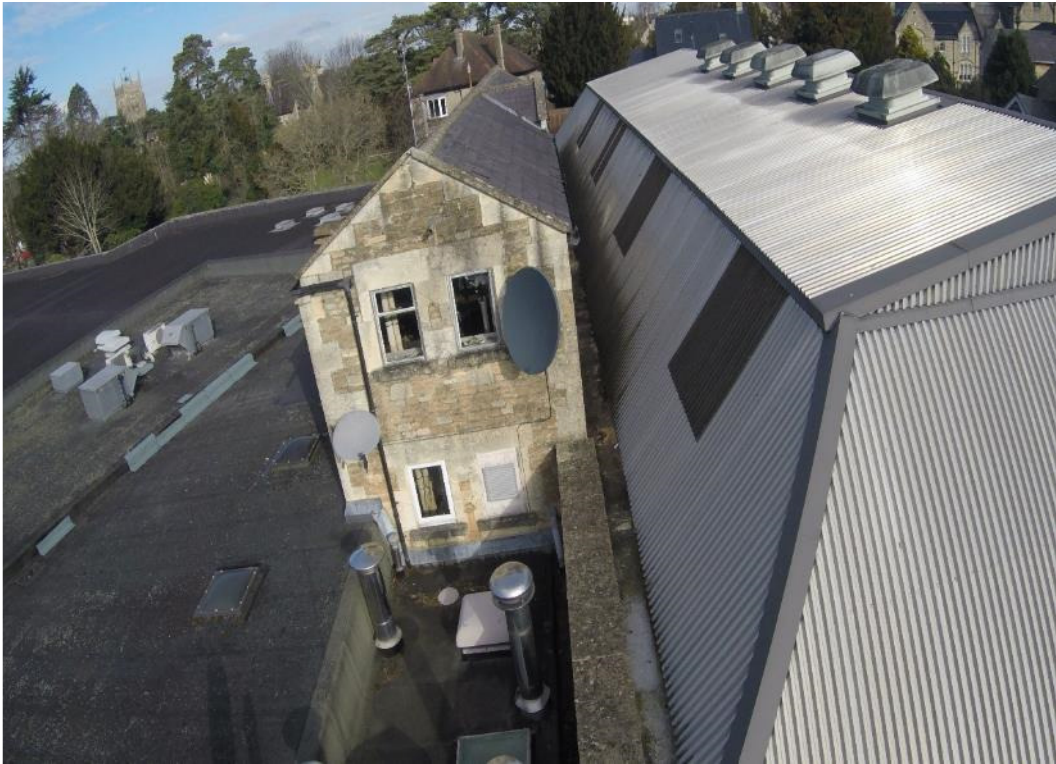
Photograph 5: Left hand elevation of the rear three storey section.
