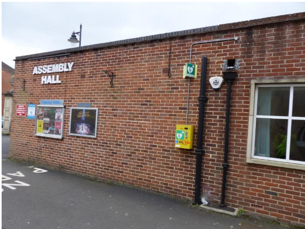
Photograph 2: Left hand side of the front elevation
