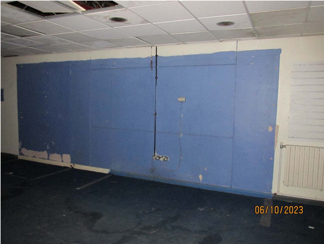
Location in existing Foyer of infilled opening to the Assembly Hall
