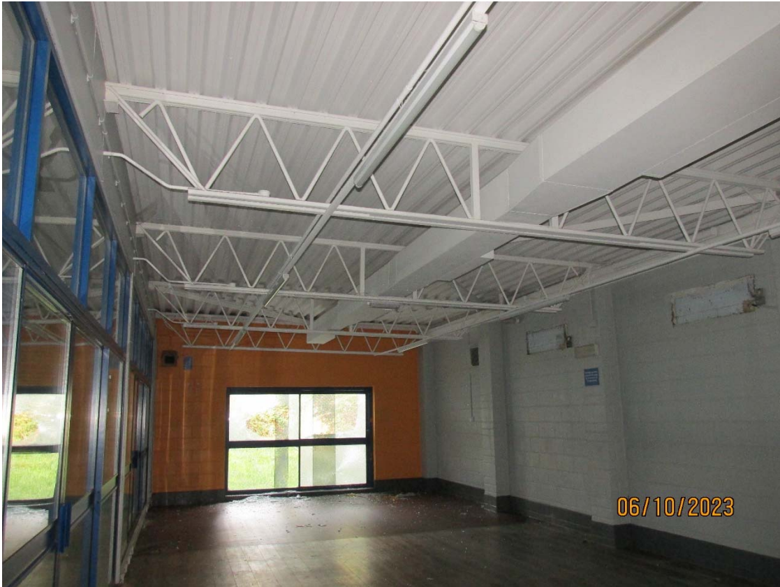
Roof structure above the Fitness Suite
