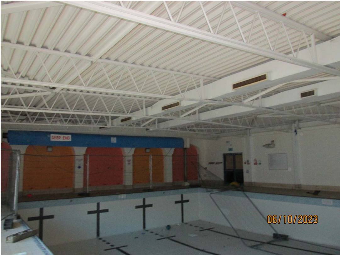
Roof structure above the Swimming Pool
