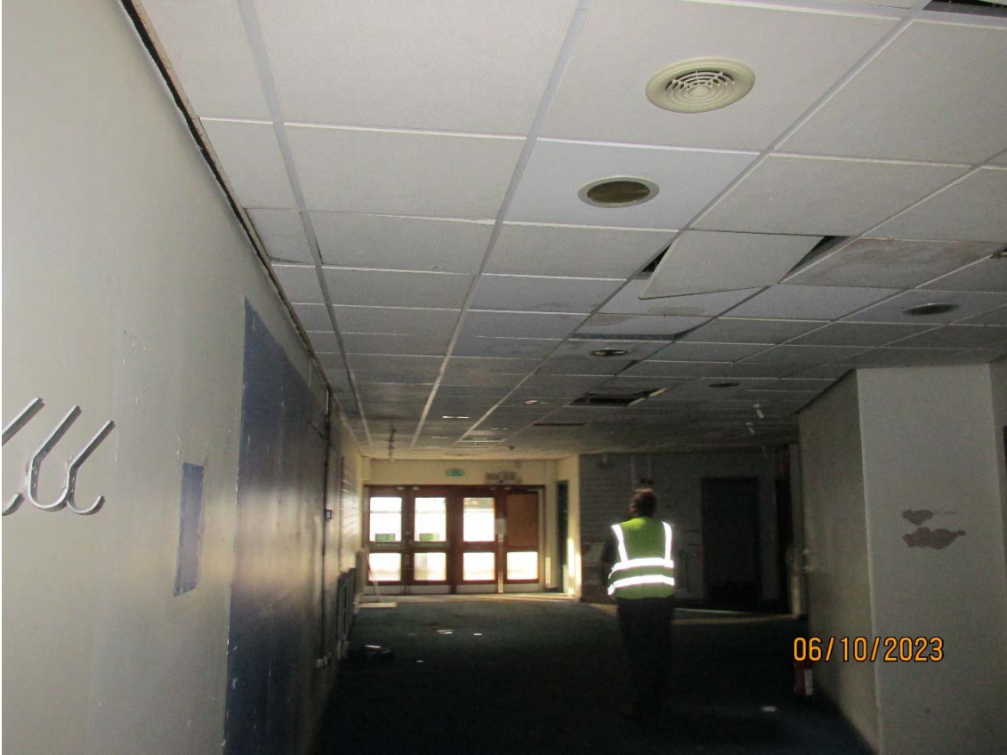
Existing Foyer with suspended ceiling
