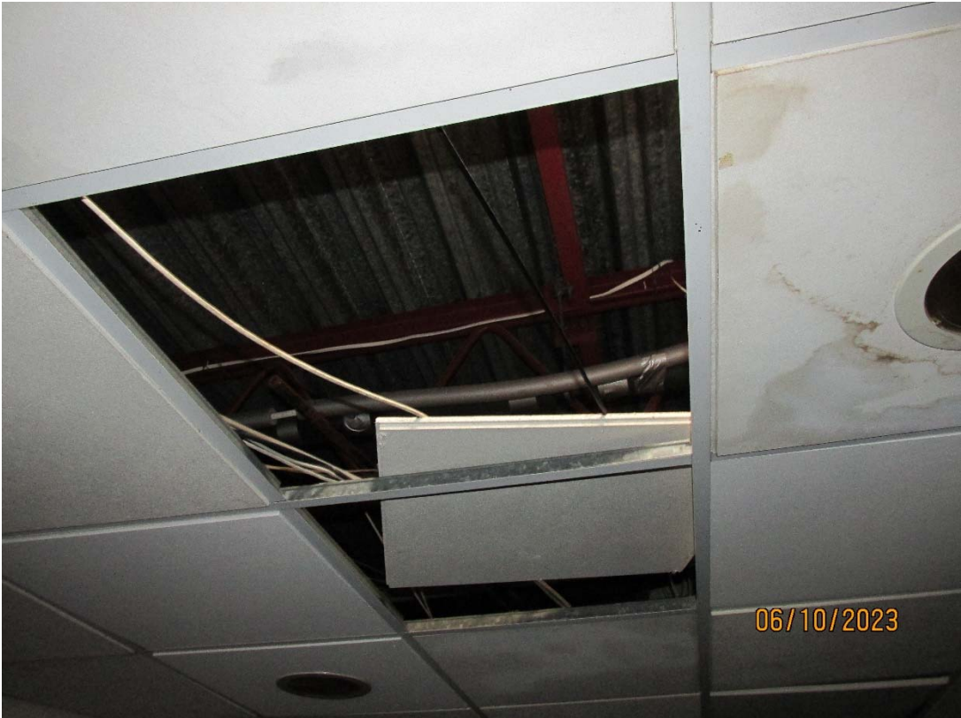
Roof structure above suspended ceiling in Foyer
