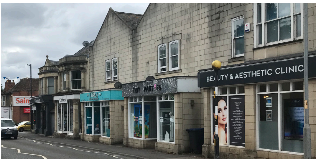
Figure 25: Consistent, but tired shopfronts, Bath Rd
