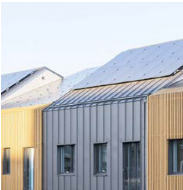
Figure 52: PV cells on pitched roof
