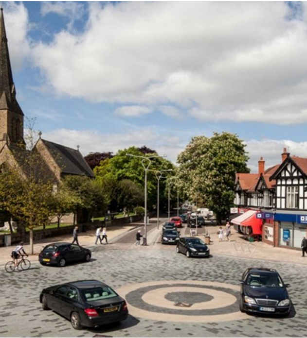
Figure 53: Distinctive materials for junction, footpath, use of shared surface for all users to reduce traffic speed in Poynton
