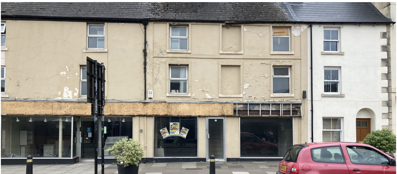
Figure 92: Vacant units, Lowbourn
