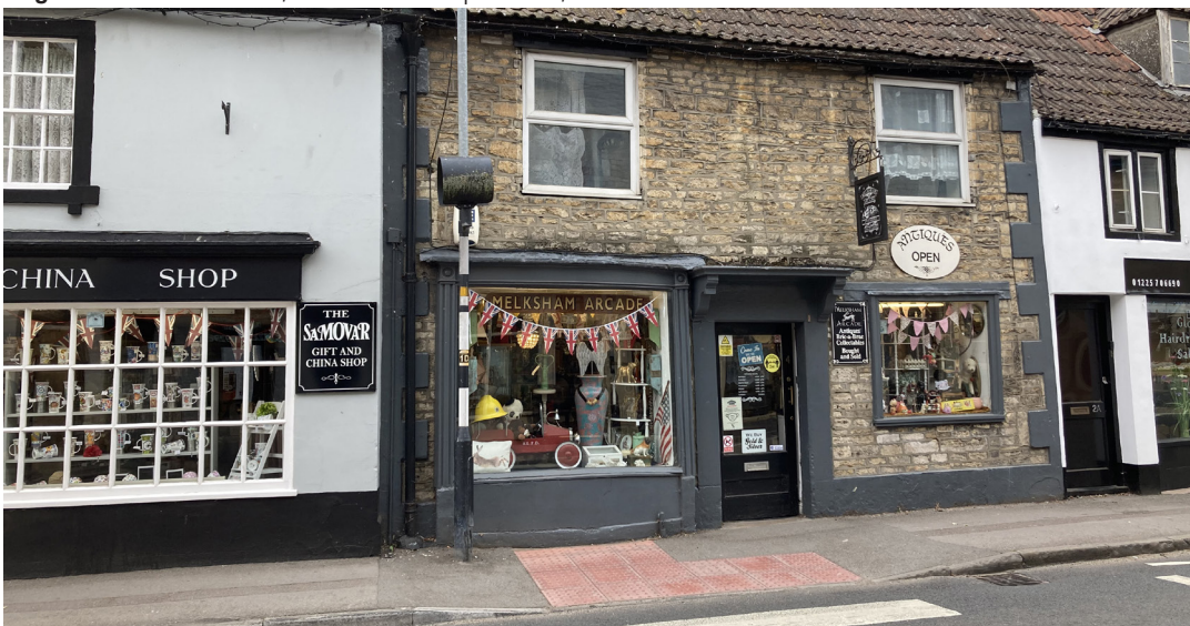
Figure 26: High quality shopfronts, Church St
