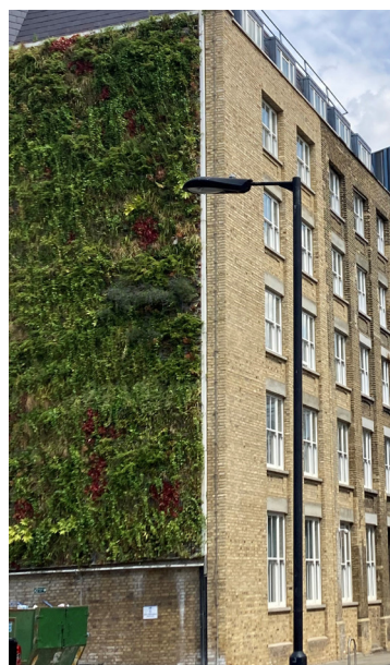
Figure 48: Living wall, London
