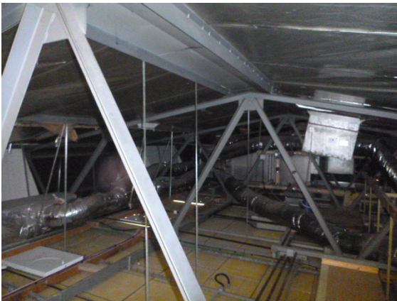
35. View across the Assembly Hall roof void steel trusses.
