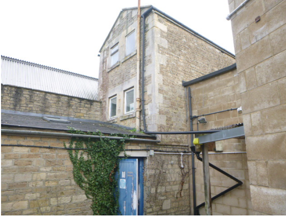
19. Rear arrangement with older redundant stone central core above.
