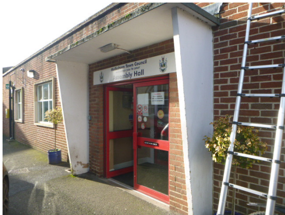
5. Main front door with level access.
