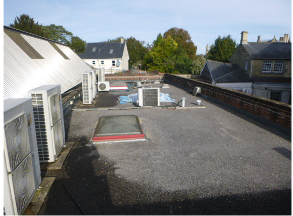
14. View across the flat roofs serving the frontage.
