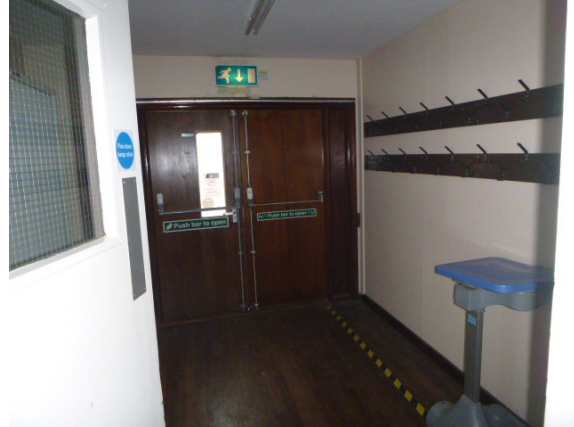
26. View of a typical fire exit route to the side escape.
