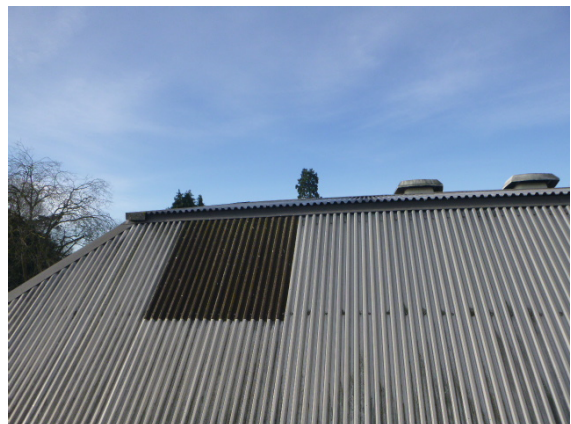
24. GRP roof light to the metal clad roof.
