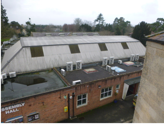
1. Front elevated view of the Assembly Hall and roofs.
