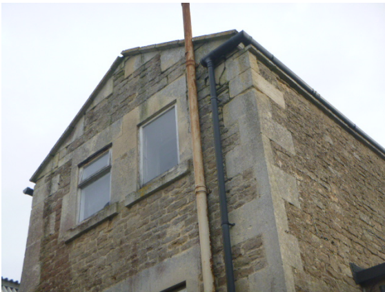
21. Indication of the older core building. New gutters and roof covering.
